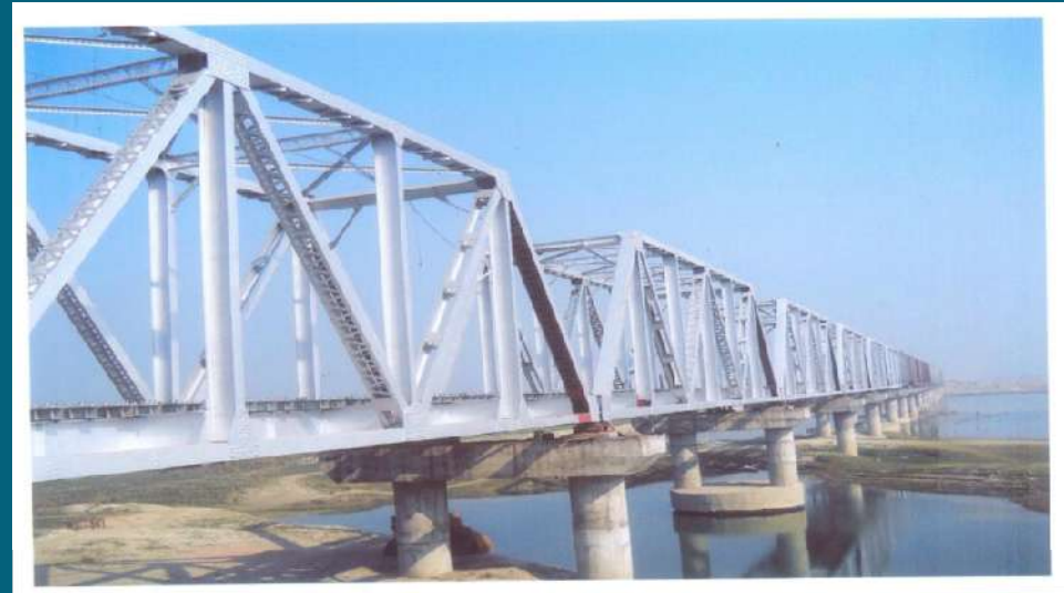
Launching &Erection of 4 nos OWG 74 mtr span over River Ganga ROB
