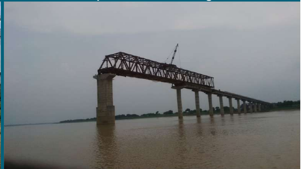
Launching &Erection of 4 nos OWG 74 mtr span over River Ganga ROB
