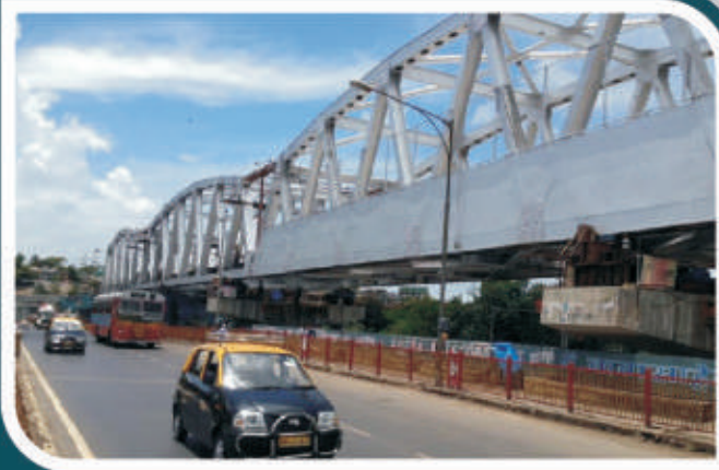
3 Nos OWG For Mumbai Monorail Project, L&T
