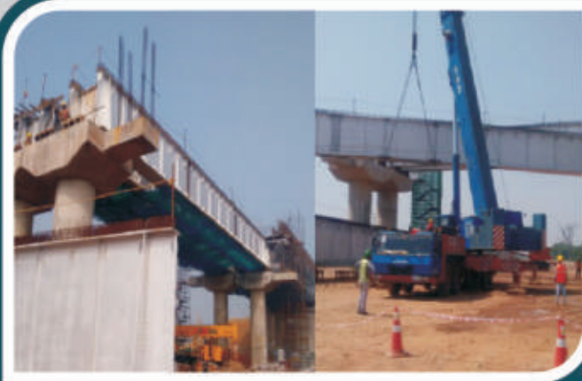
Erection of Girders for DFCCIL Tata Projects Ltd
