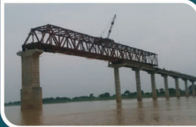
Launching & Erection of 4 nos OWG 74 mtr span over River Ganga ROB
