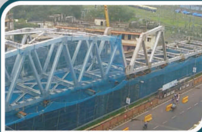
3 Nos. of Open Web Girders for Mumbai Monorail Project (L&T)
